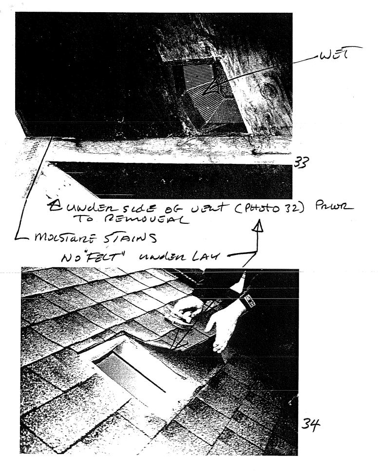
UNIT#57 WATER SIJTURATED UNDER SIDE OF DECK
