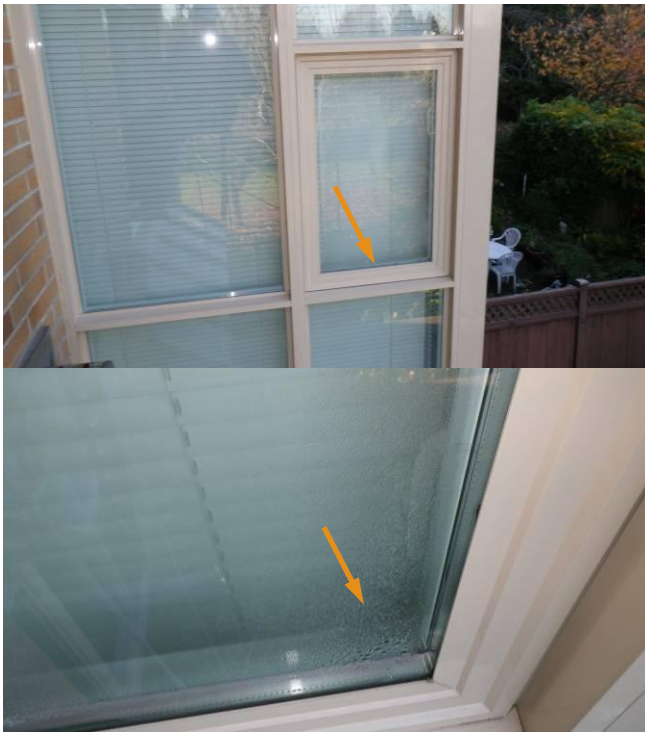
Fig. 2.2.2 Failed insulating glass unit on the 2 nd floor, east elevation.
