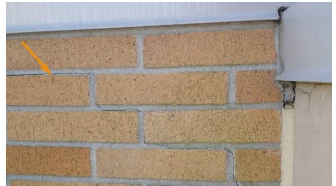
Fig. 2.1.5 Localized cracking of the brick masonry mortar joints on the 10th floor, northeast corner (north facing).
