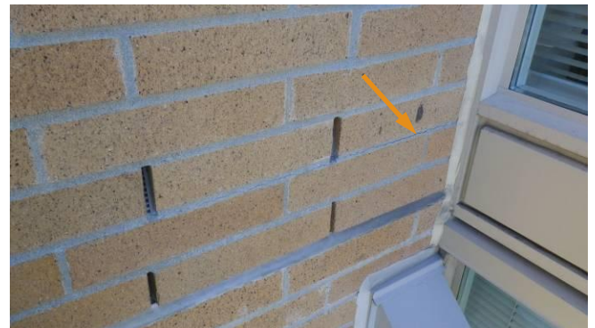
Fig. 2.1.6 Localized cracking of the brick masonry mortar joints on the 4 th floor, west elevation.
