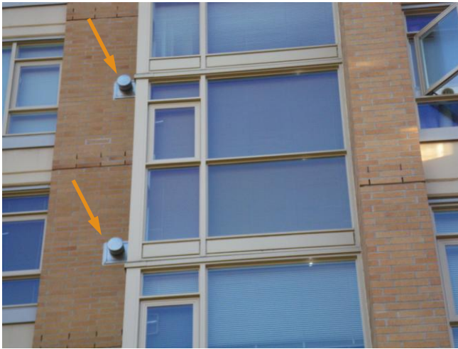
Fig. 2.2.2.8 Typical stainless steel fireplace exhaust vents, west elevation.
