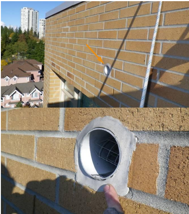
Fig. 2.1.7 Sealant cracking at the roof overflow to brick masonry veneer interface, west elevation.
