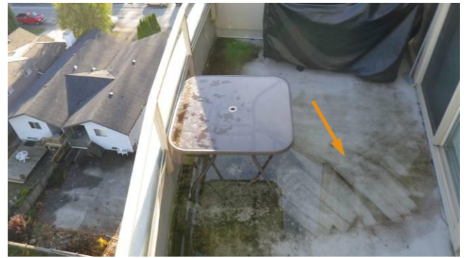
Fig. 2.3.2 Minor water ponding at Suite 1004.
