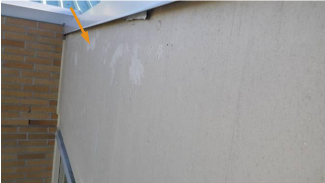
Fig. 2.1.2 Elastomeric paint on concrete wall is scuffed, east elevation.
