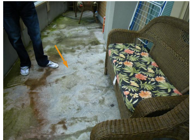
Fig. 2.3.4 A cement topping was applied over the traffic coating, Suite 1003.
