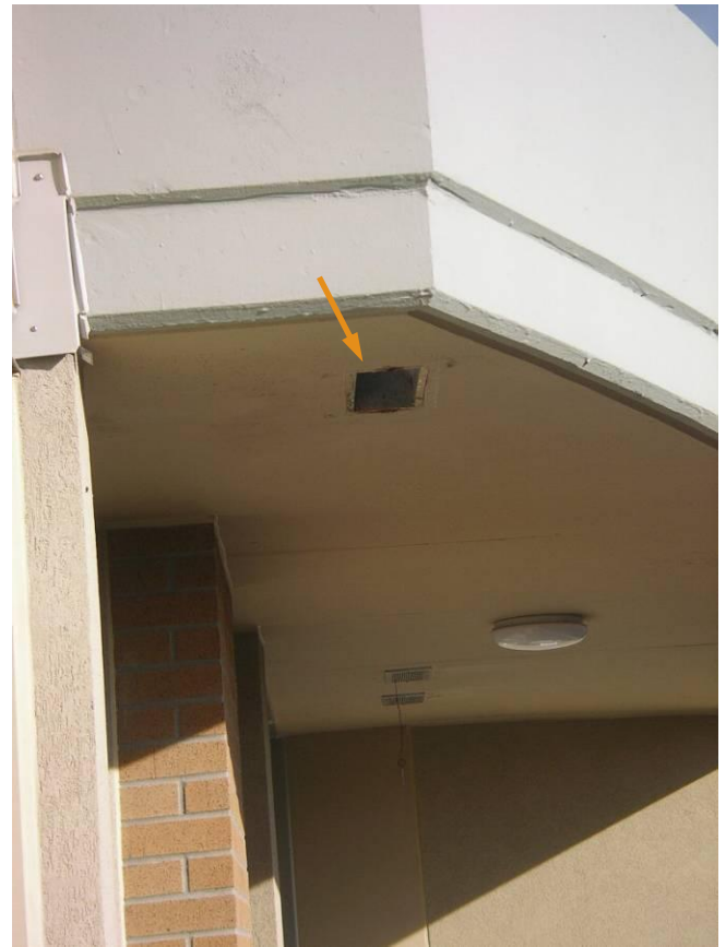
Fig. 2.2.2.9 Missing exhaust grill from in-slab discharge vents on the 5 th and the 8 th floors, south elevation.
