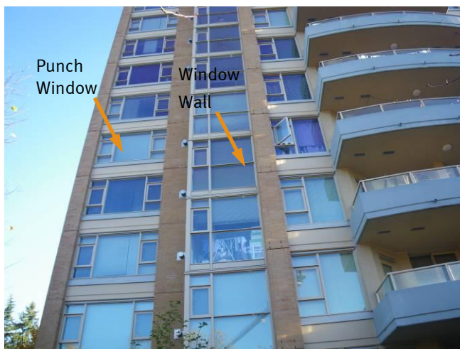
Fig. 2.2.1 Window wall and punch window on west elevation.
