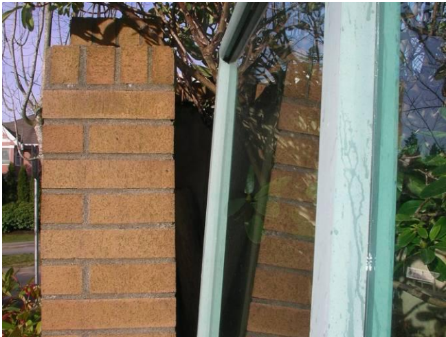
Fig. 2.5.2 The west-facing patio guardrail at Suite 101 is not adequately secured to the brick masonry.
