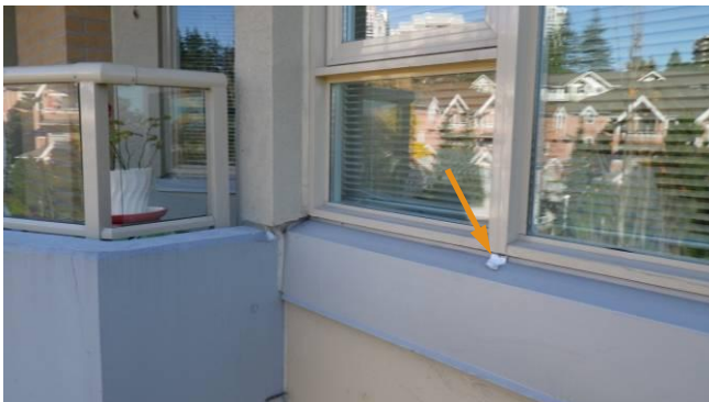
Fig. 2.2.4 Identification labels were not removed prior to sealant installation at various window sections.
