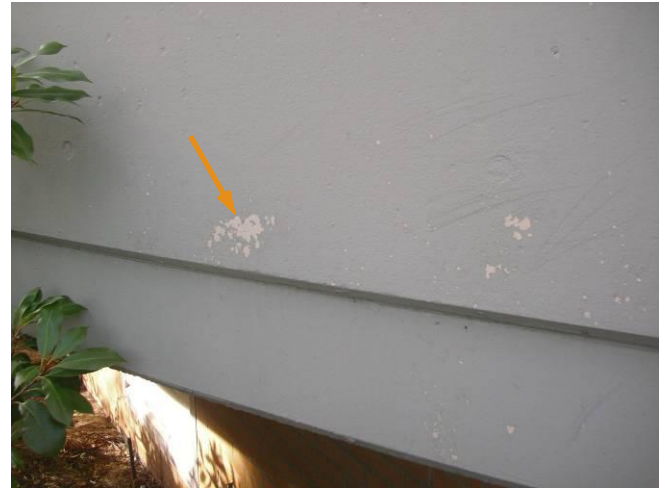
Fig. 2.3.3 Minor damage to exterior coating on exterior face of balcony on level 1, south elevation.
