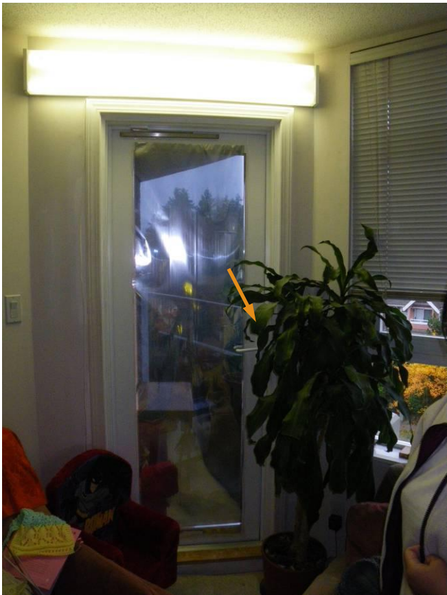
Fig. 2.2.7 The swing door is hard to operate, Suite 606.
