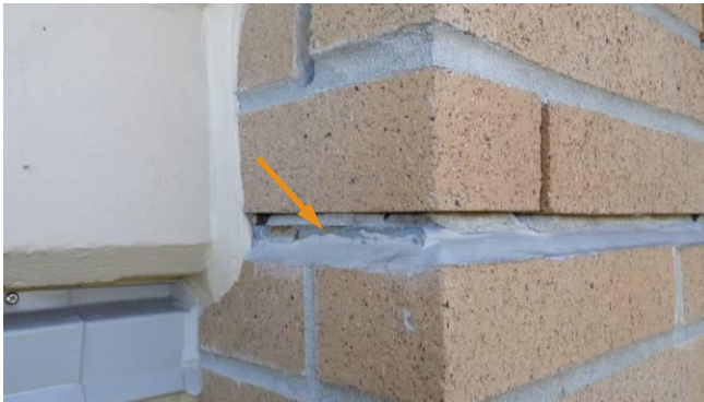
Fig. 2.1.8 Discontinuous sealant at the shelf angle, east elevation of the 10 th floor.
