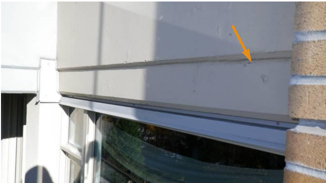
Fig. 2.1.3 Sealant cracking at concrete cold joint on the 5 th floor, west elevation.
